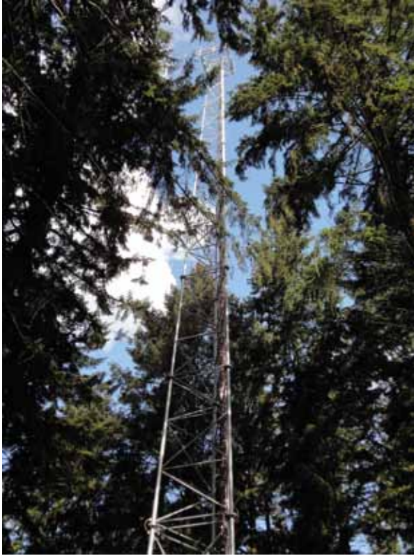
Tower for Eddy Covariance turbulent flux measurements at a mixed forest site at Vielsalm, Belgium.
